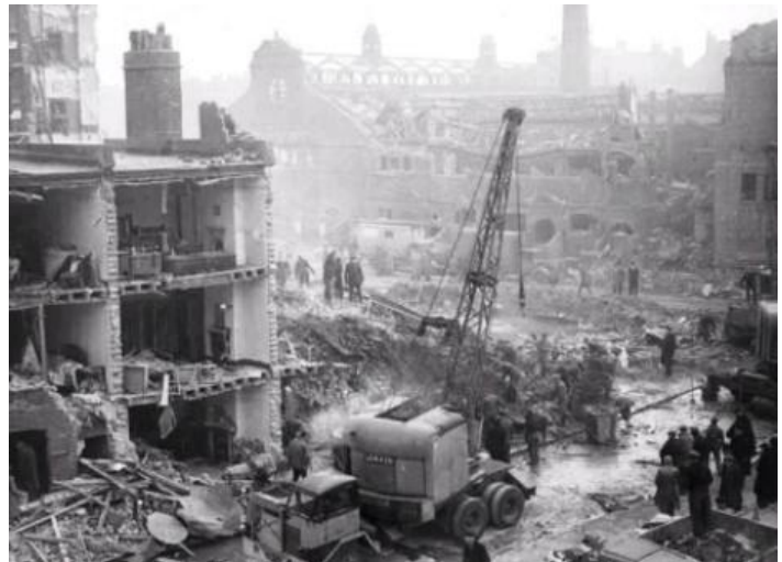
Lambeth North, London, 1944. Photograph from internet not part of original story.
